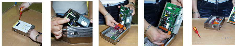
Fig. 28: Replacing a controller
